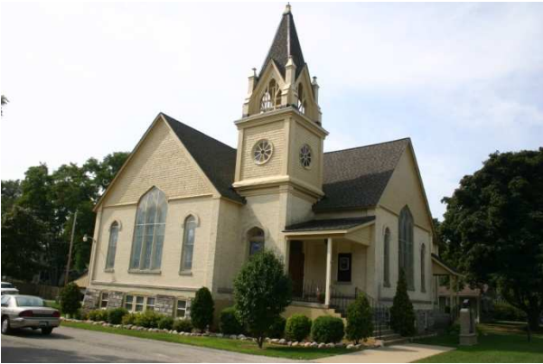
ERUM, Sept. 2011, Corner View- East Façade
