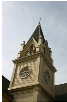
ERUM, Sept. 2011, Steeple in northeast corner
