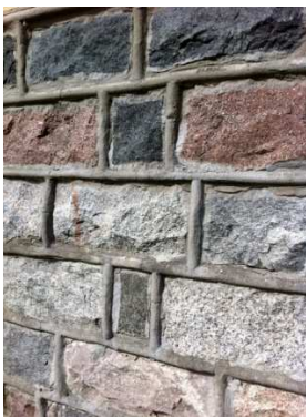
ERUM, Sept. 2011, Foundation on North façade, northeast corner
