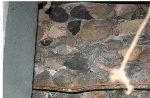
ERUM, Sept. 11, EXTERIOR WALL OF FURNACE ROOM
